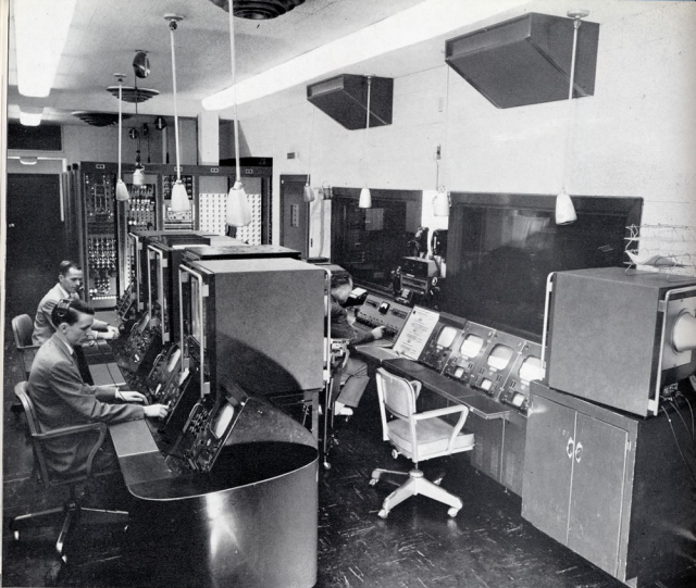
FIG. 15. WBTV's main control room. Master audio and video switching facilities are concentrated in the low console at the right (just in front of the windows which look into the announcers' booths and the studios). Camera control operations are performed at the console, at the left, which contains controls and monitors for all live cameras, film cameras, and Chromascan units. Equipment racks are located at the two ends of the control room. The floor plan of this control room is shown in Fig. 16, on the opposite page.
