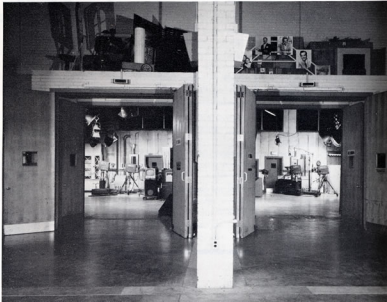
FIG. 12. The doors from the prop area into the studios are ten feet high by ten feet wide. There are two sets of doors to each studio with a "sound lock" between. This keeps noise from the prop area from getting into the studios during programs.
