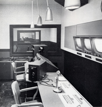
FIG. 22. TV studio control booths and clients' booths are arranged in a line on second floor (see Fig. 9, Pg. 38). Director sits at near position, does his own switching. This view is from TV-1 control room and looks through three double-glazed windows into TV-2 control room 74 feet away.
