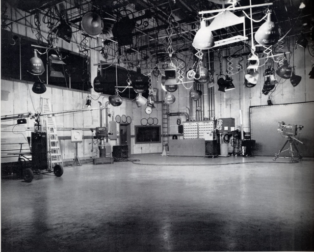
FIG. 7. WBTB's Studio TV-2 is 40 feet by 60 feet, has a ceiling height of 27 feet. Windows of clients' booths and control booths on second floor are at top left. Window of announcer's booth is in center, with lighting control board just to the right of it. Both studios have "prestressed, post-tensioned" concrete floors poured as single slabs. Walls and ceiling are covered with two-inch thick, rock-wool blanket. Outlets are provided in the two studios for both monochrome and color cameras.
