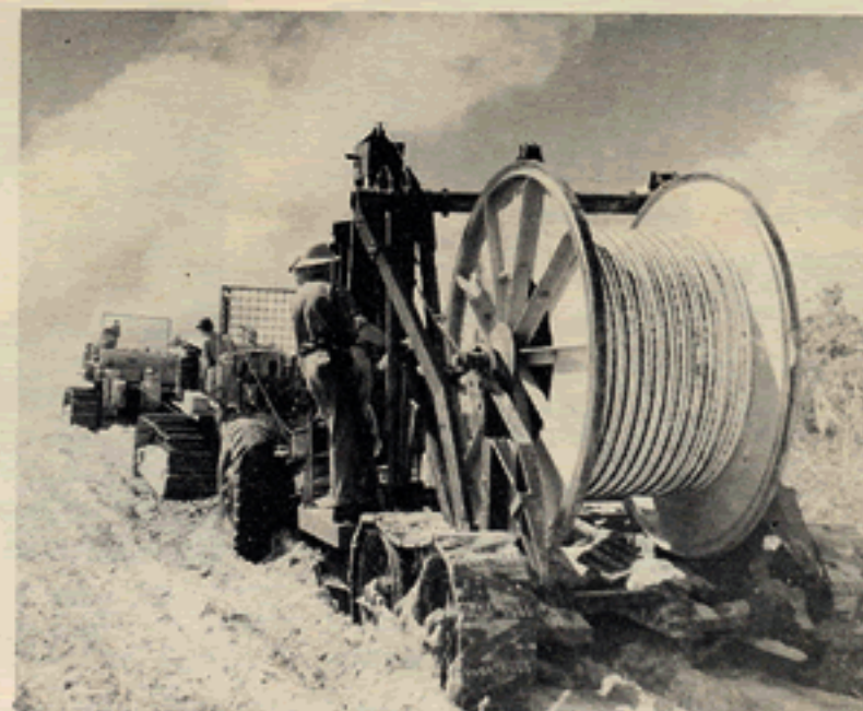
Laying the coaxial cable.
